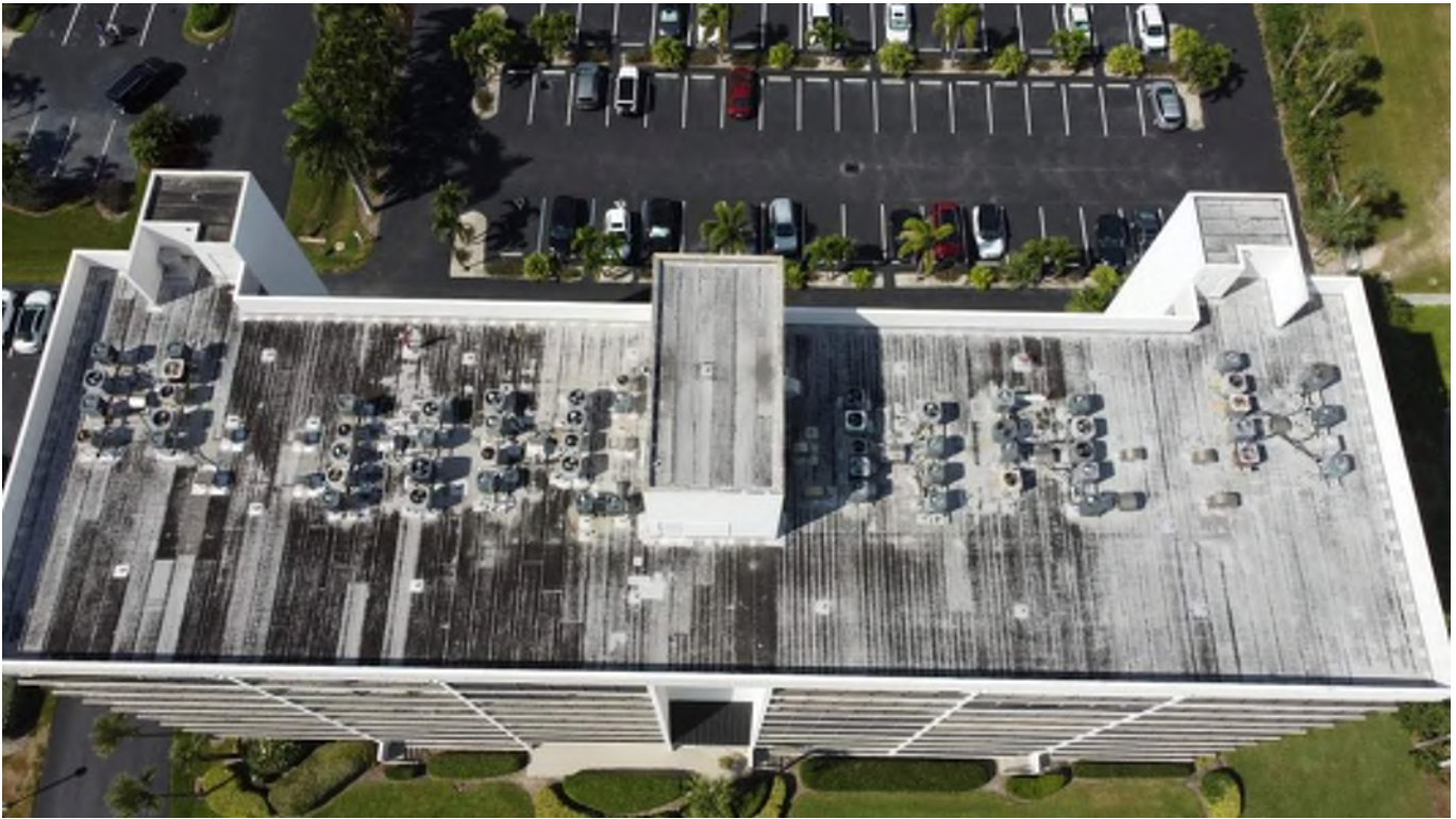
5061 N A1A (Building A) – Roof
