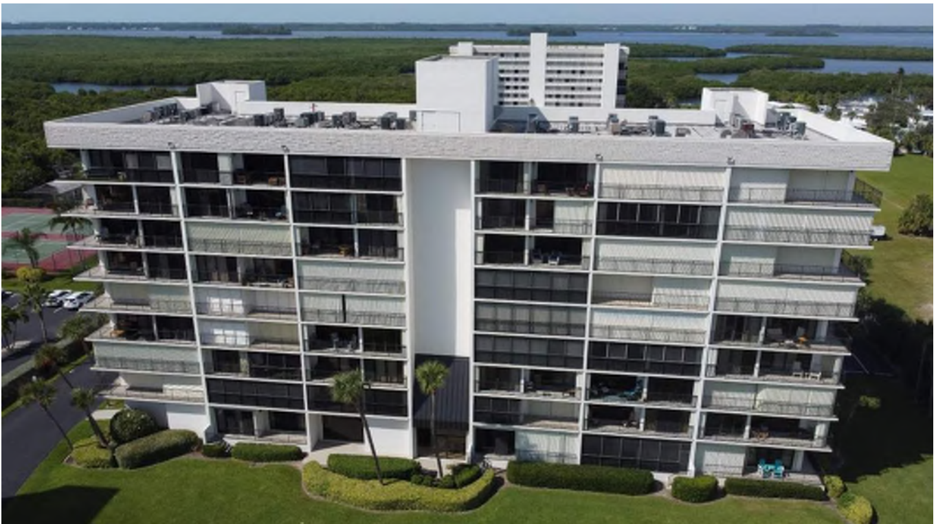
5061 N A1A (Building A) – East Elevation
