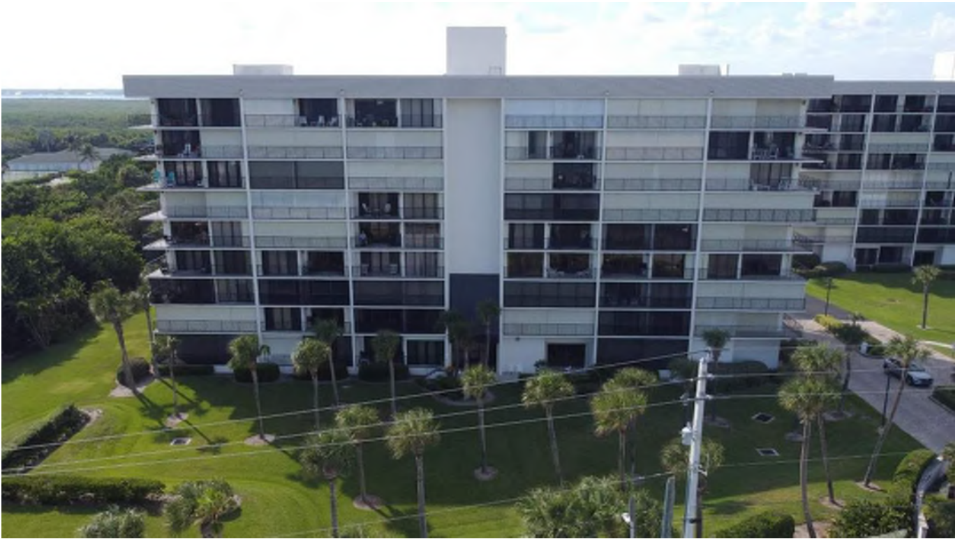
5059 N A1A (Building B) – East Elevation
