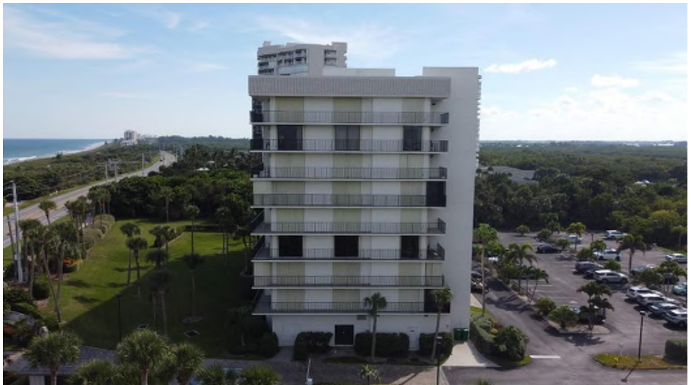
5059 N A1A (Building B) – North Elevation
