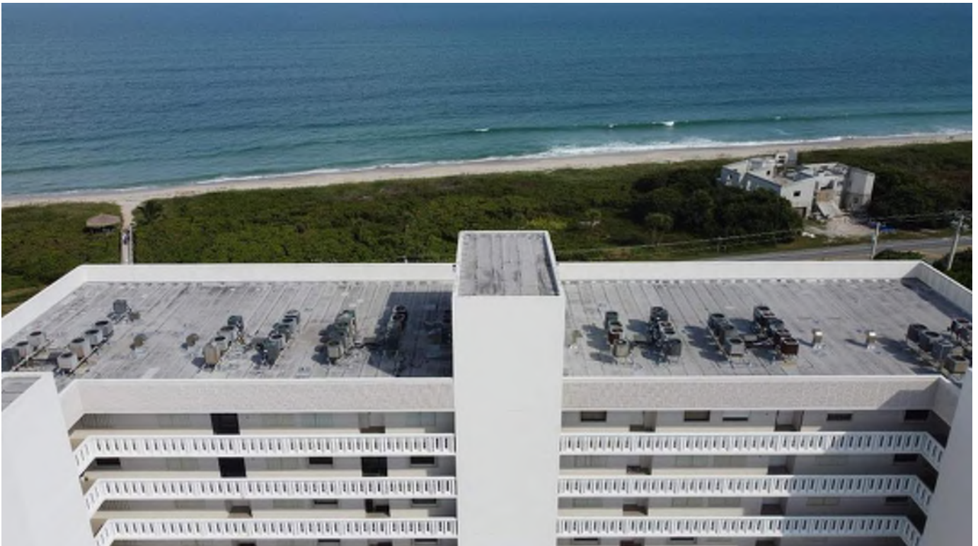
5059 N A1A (Building B) – Roof
