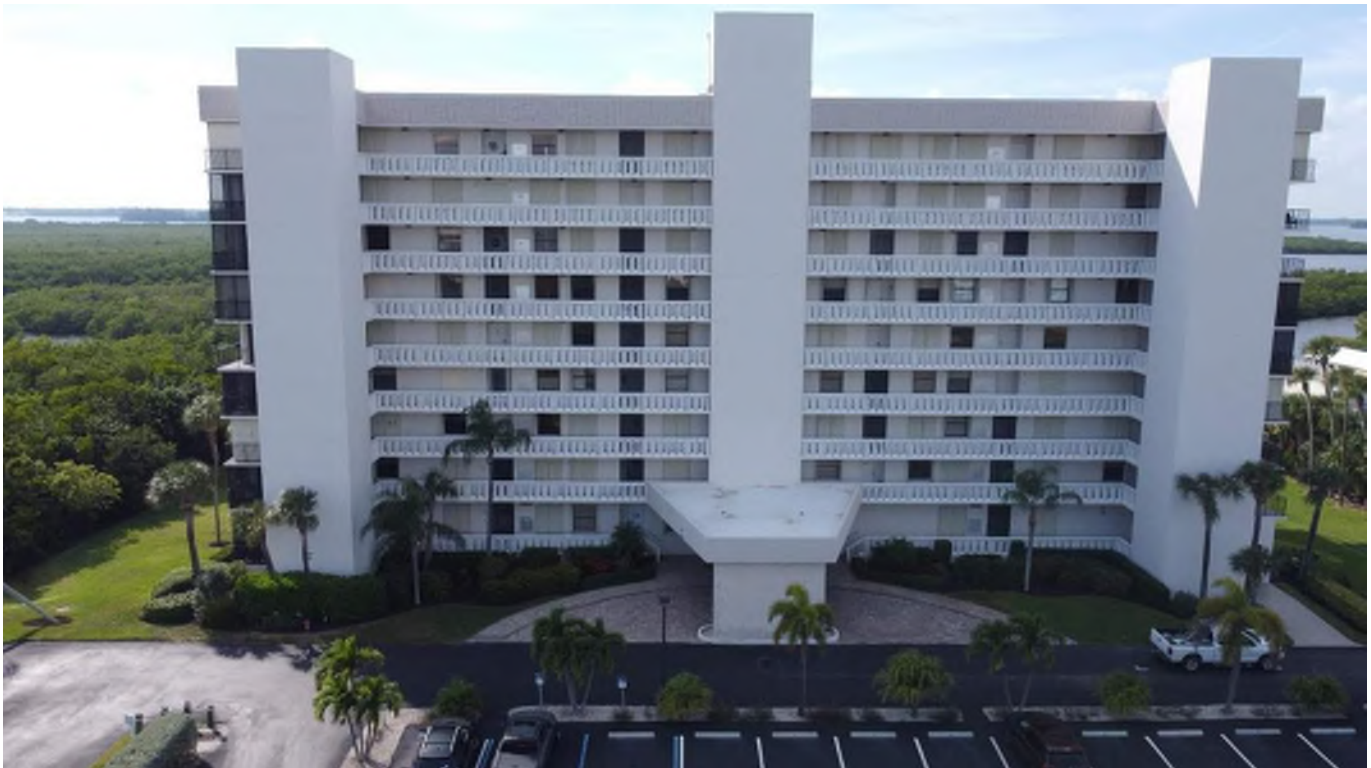
5055 N A1A (Building C) – East Elevation
