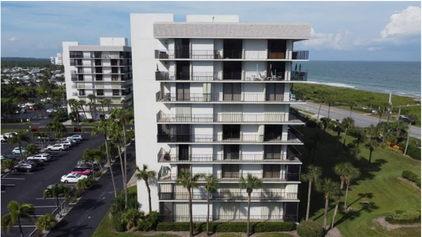
5059 N A1A (Building B) – South Elevation
