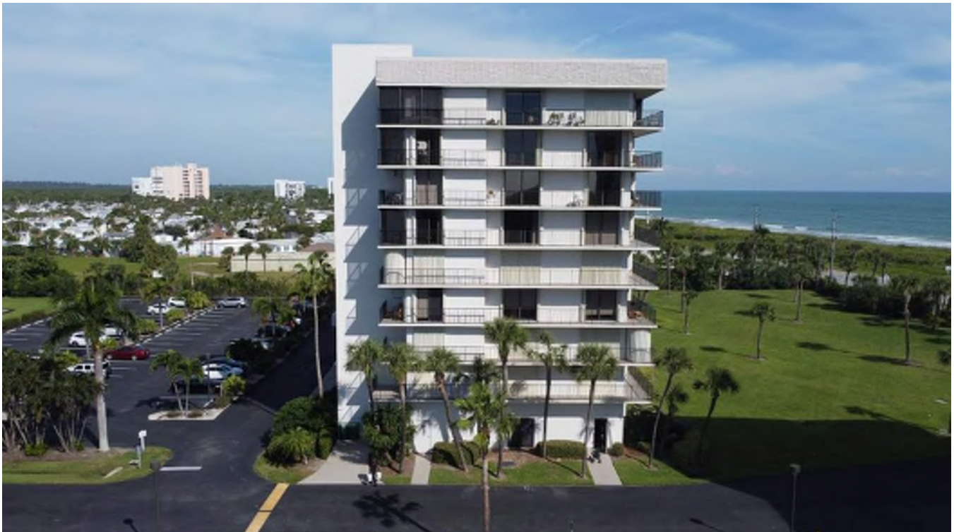
5061 N A1A (Building A) – South Elevation
