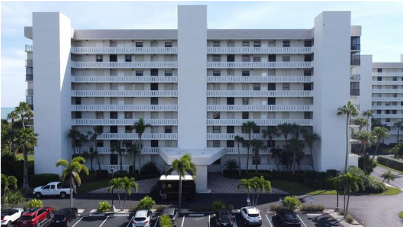
5061 N A1A (Building A) – West Elevation
