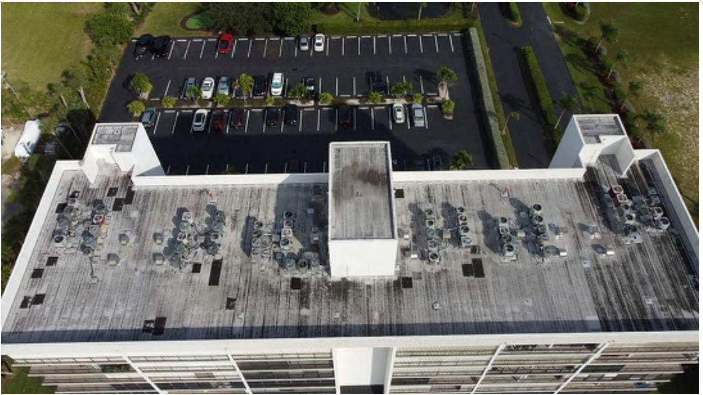
5055 N A1A (Building C) – Roof
