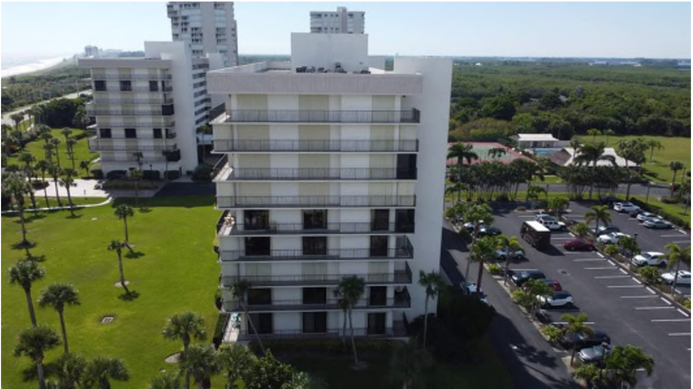
5061 N A1A (Building A) – North Elevation
