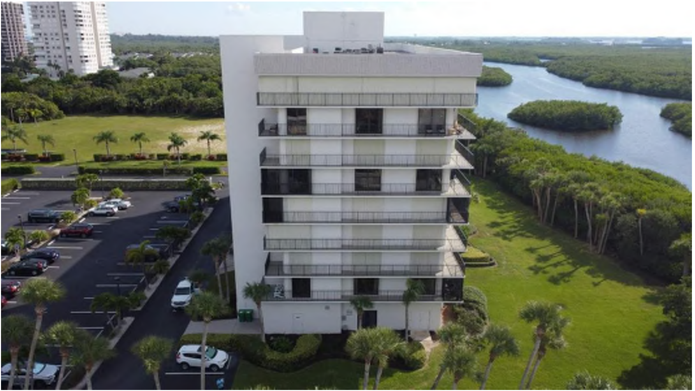
5055 N A1A (Building C) – North Elevation
